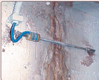
• Model 4420 Crackmeter installation.
